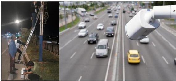
Figure 1. The process of installing measuring cameras to study the amount of traffic flow
