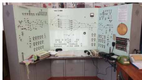
2-rasm. Tablo turi 1A1B1V1C-II releli va marshrut – releli markazlashtirish pulti
