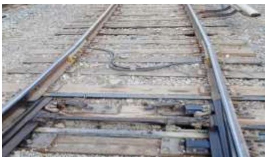
4-rasm. Yeterli donadorlikka ega bo'lmagan metropoliten yo'llarining ballast prizmasi
